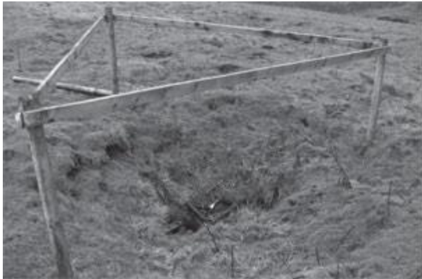
Plate 5.0 An inadequate method used to secure an abandoned mine entrance
